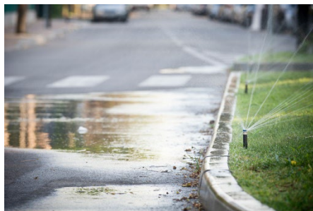
Wasteful overspray due to poor irrigation design and maintenance
