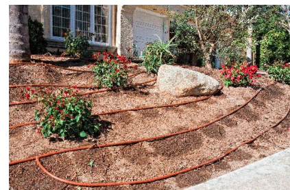
On-surface dripline installed in typical grid layout provides low volume irrigation to plants without overspray
