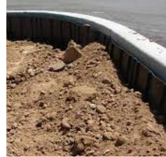
Tree root barrier at parking lot planter
